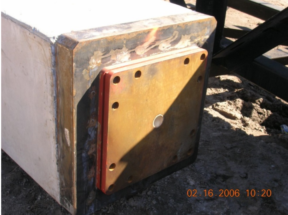
Male portion on upper pile section.
