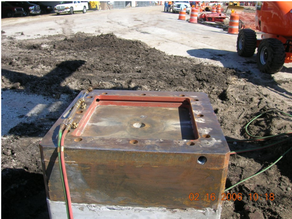
Female portion on lower driven section.
