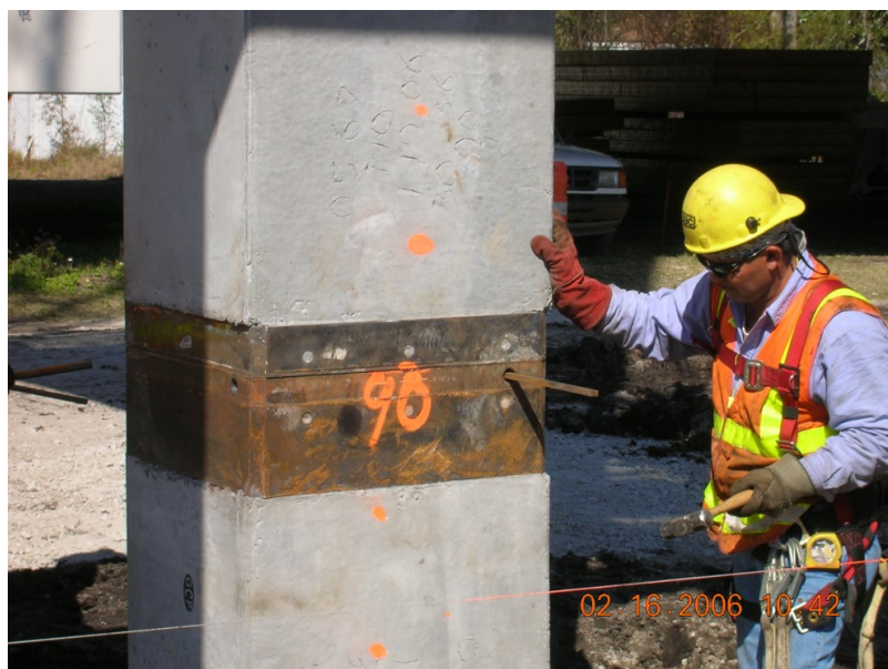
Drive square pins and all four corners with a 5lb sledge hammer.
