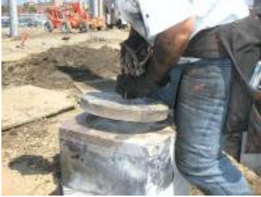
Removing the Drive Plate
