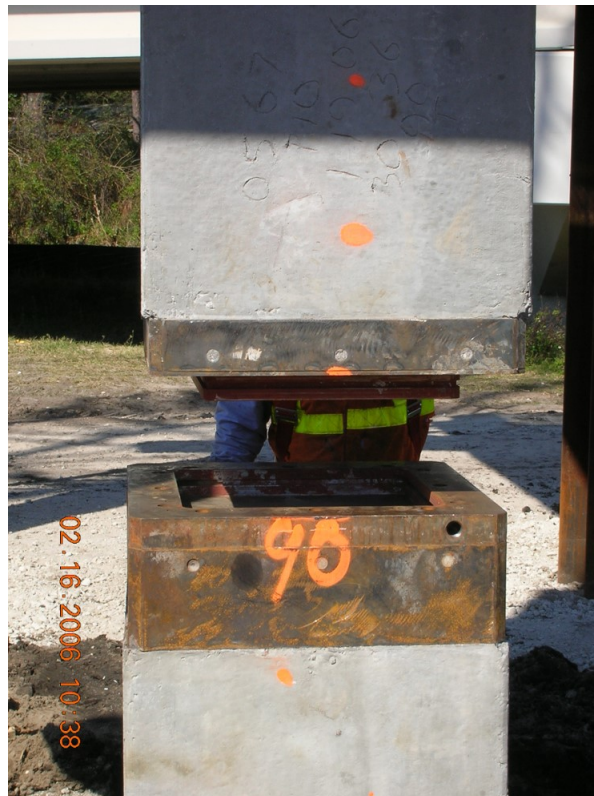
Lower upper pile section onto already driven lower section.
